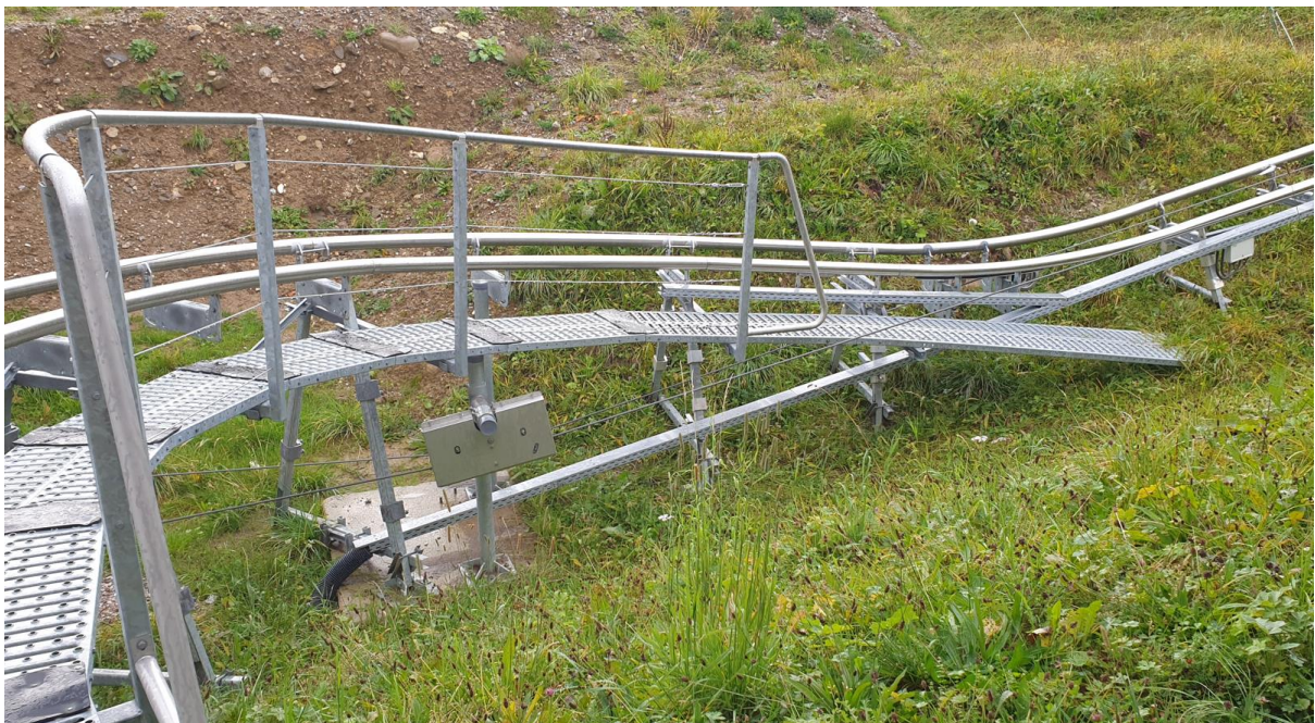
Figure 7: Example walkway with a ramp (can be a ladder) to ground level
