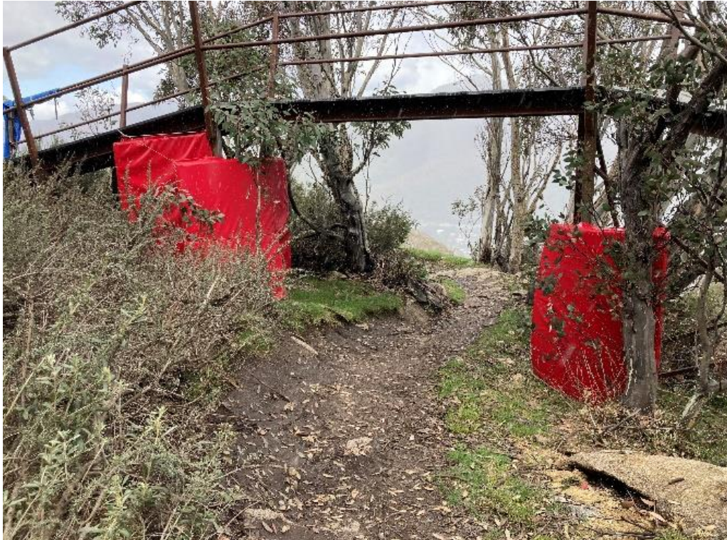
Figure 12: Example of padding installed on posts within proximity of MTB Trail Overpass
