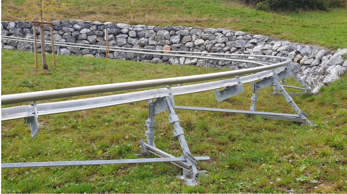
Figure 3: Example trestle supports on a bend
