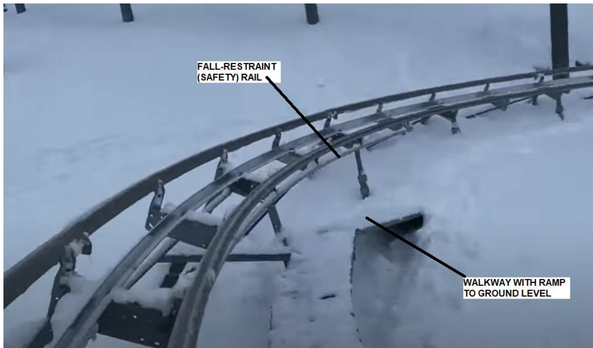
Figure 8: Downhill track with walkway, safety rail and ramp
