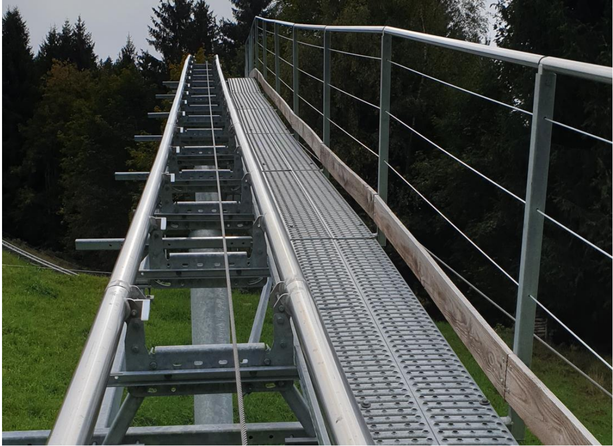
Figure 6: Example of uphill track walkway and handrail
