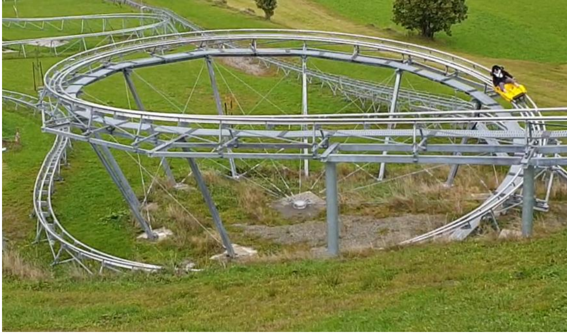
Figure 5: Example of bracing rods within a track circle
