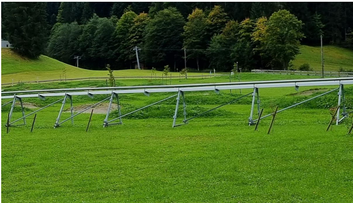
Figure 4: Example trestle supports on straight track
